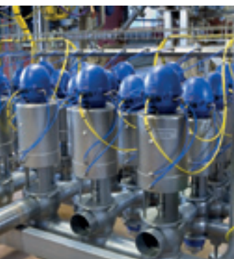
Complete flow battery at protein processing plant, Germany
