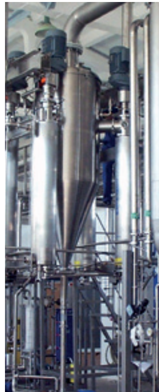
Scraped-surface evaporator system for viscous food, USA
