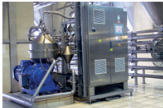
Complete system for beer recovery from tank bottoms, Romania
