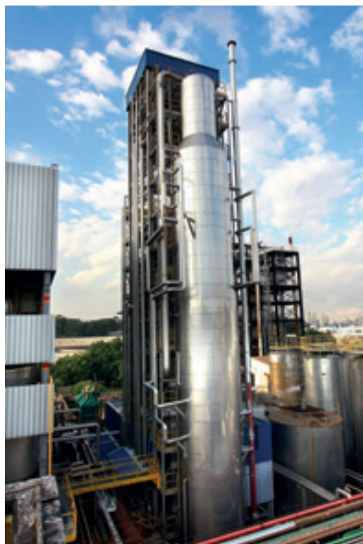
Semi-continuous deodorization system for vegetable oil, Brazil
