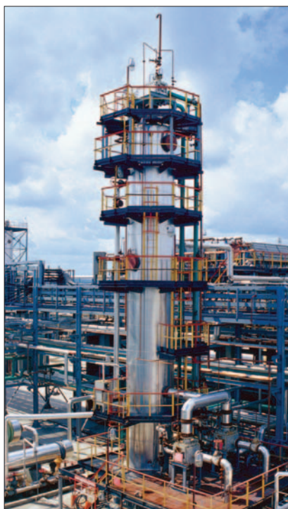
Syzran refinery MEA stripping tower, with twin Compabloc reboilers at the base of the column and a Compabloc reflux condenser atop it.
