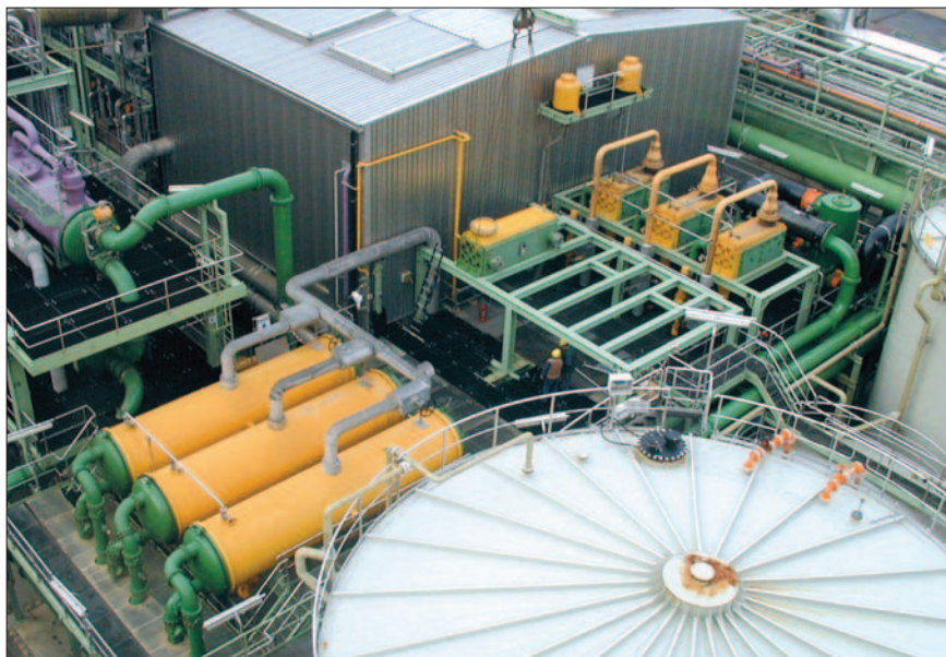
The three Compabloc units on the right have half the footprint of the three shell-and-tube units on the left but 50% greater capacity!
