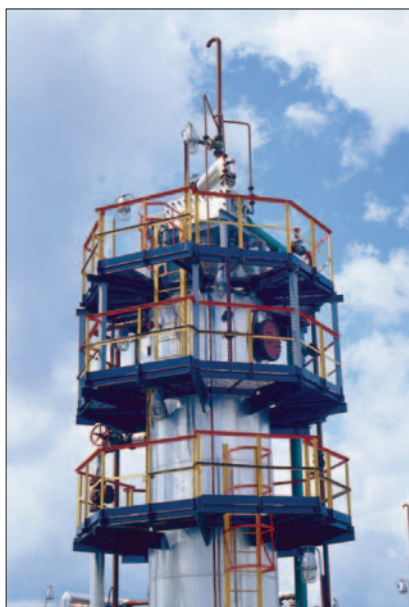
Detail of column-mounted reflux condenser.
